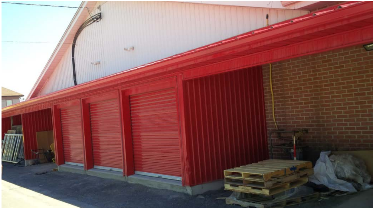
Figure 5: Rear Façade at 22 Ottawa Street West, Havelock
