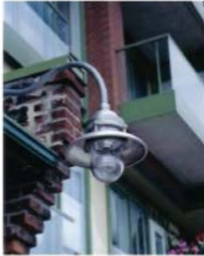
Traditional 'yard' style light with modern updates such as dark sky compliance rating and light shields
