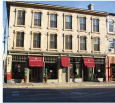
Fixed canvas awnings - highlights both entrances. note: old building with new materials in keeping with historic charac-
